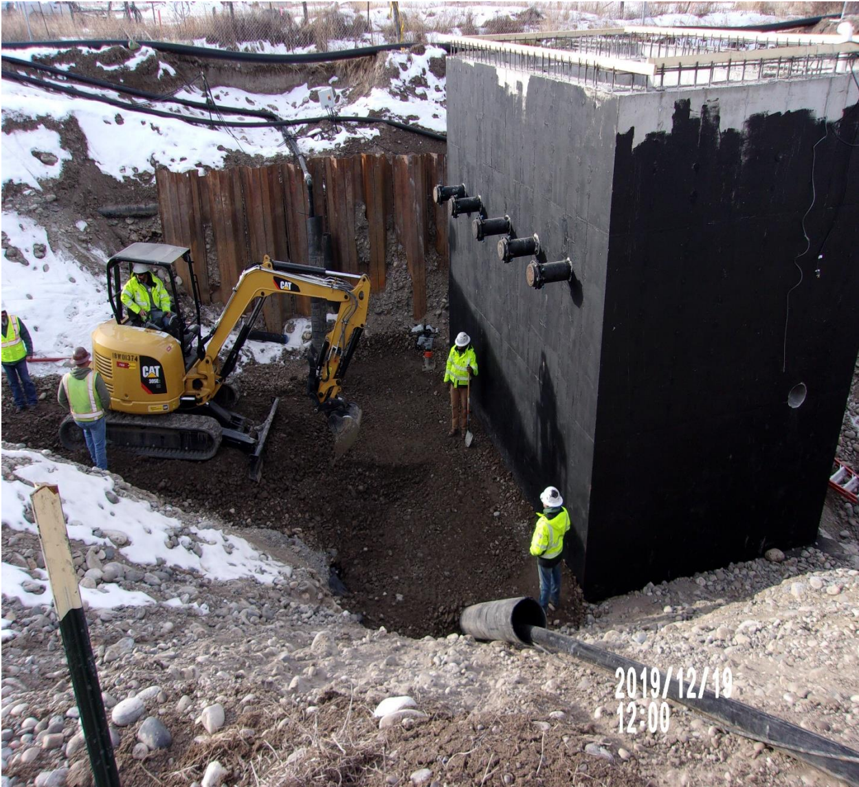
Leak test completed on Influent Pump Station, damp-proofing completed, and backfilling started.
