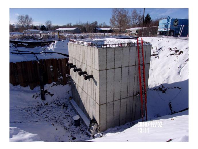
This structure will receive all of the wastewater from the district except from the Elk Grove Subdivision. The pump and control system will meter the quantity of wastewater that is processed in the new WRF or pumped to the Elk Grove Wastewater Treatment Plant for processing.
