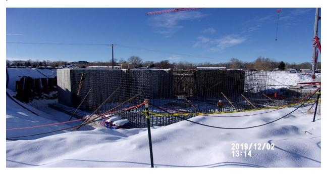
First pour of SBR #2 completed and form work going up for first pour of SBR #1.
